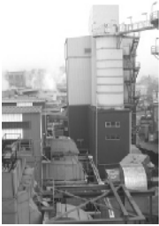
Circulating Fluidised Bed FGD Absorber with Bag Filter
